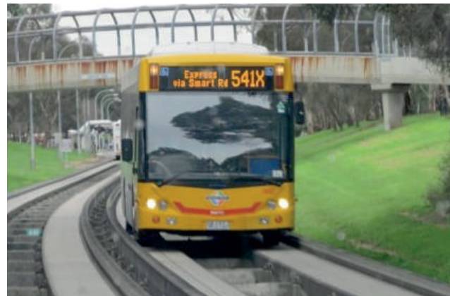
The O-Bahn bus moving around a circular section of track
